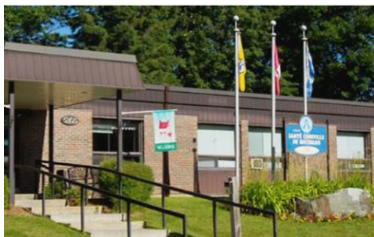
Installation de Waterloo
