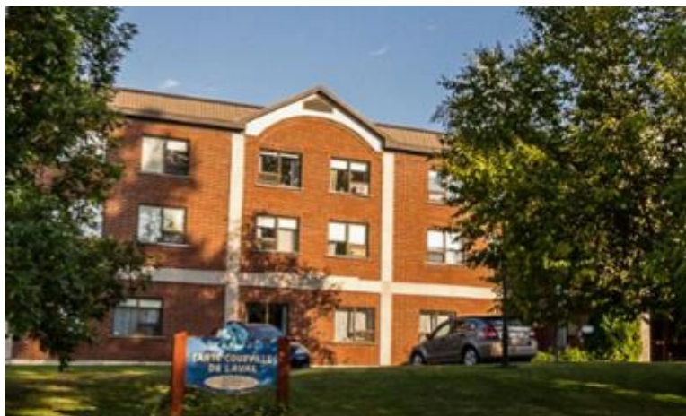
Installation de Laval
